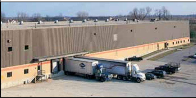
Link-Belt Parts Distribution Center
